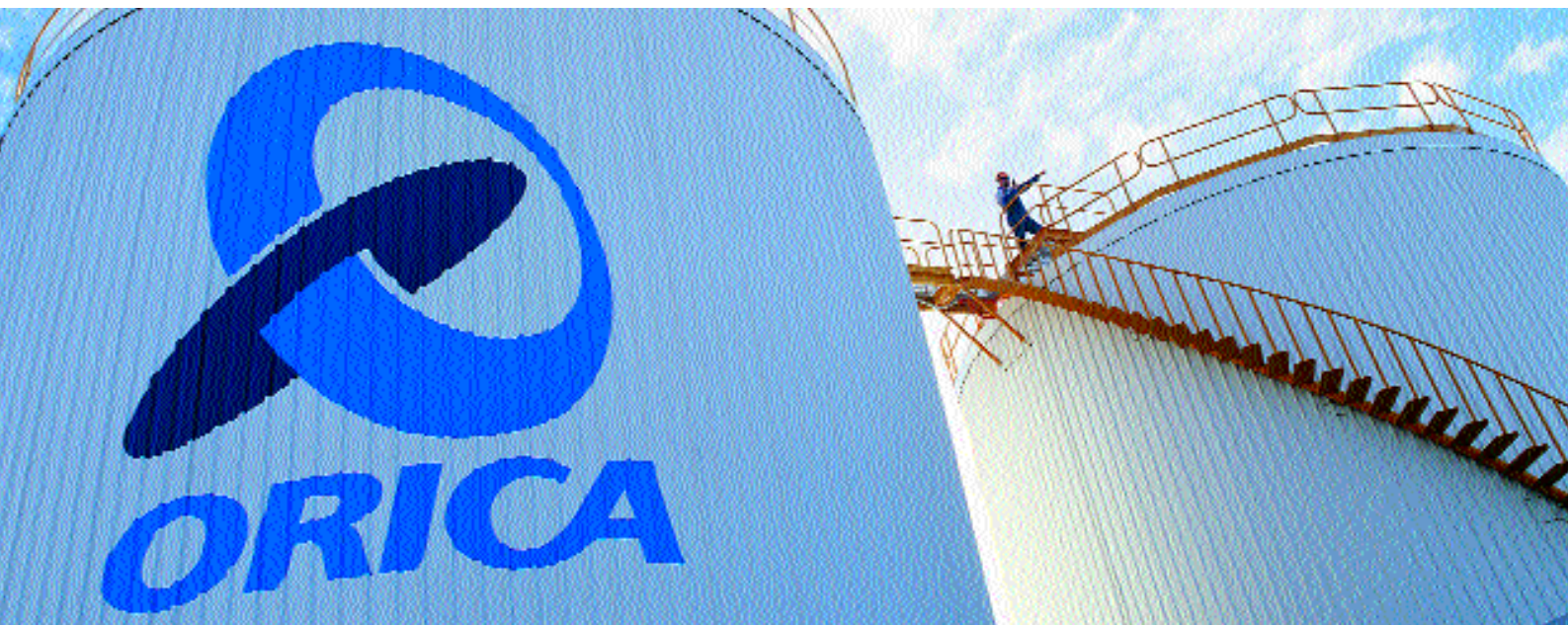
Orica Chemnet Technologies Timaru Site, South Island, New Zealand, Caustic Soda bulk storage tanks
