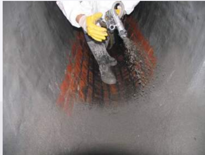
SZCZECIN sewer shotcreting
