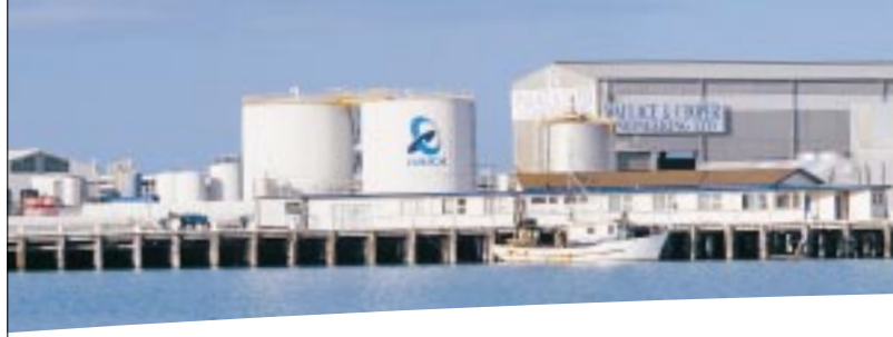
Chemicals' bulk tanker loading facility at Timaru, South Island, New Zealand
