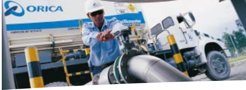
Loading a mobile manufacturing unit at the Satui (Indonesia) site
