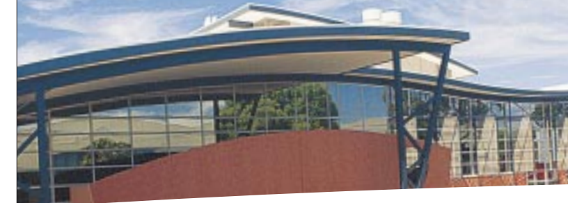
Consumer Products' new technical centre at Clayton (Victoria, Australia)
