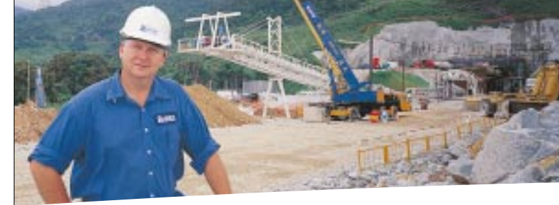
Clinton Smith at the site of one of Orica's tunnelling projects in Hong Kong
